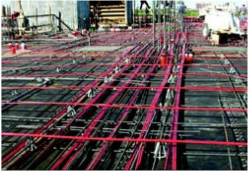
Figure 17: Two-Way PT Floor System (concreteconstruction.net)
