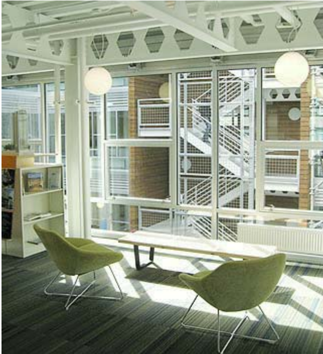
Figure 15: Exposed Castellated Beam Construction (DJC.com)
